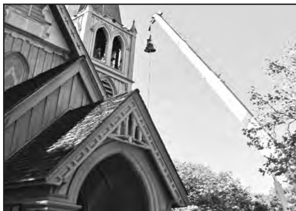
Installing the Trinity Carillon
