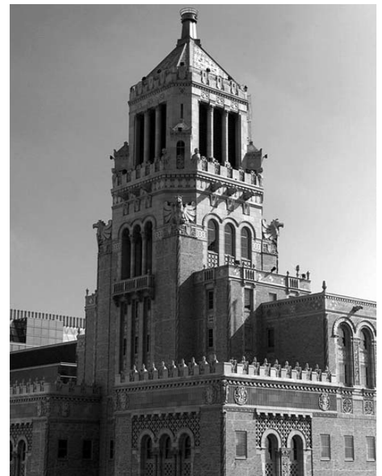
Mayo Clinic Plummer Building
