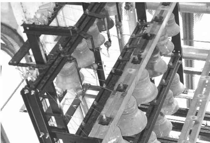
The reframed treble section showing a compact design with much shorter clapper wires
